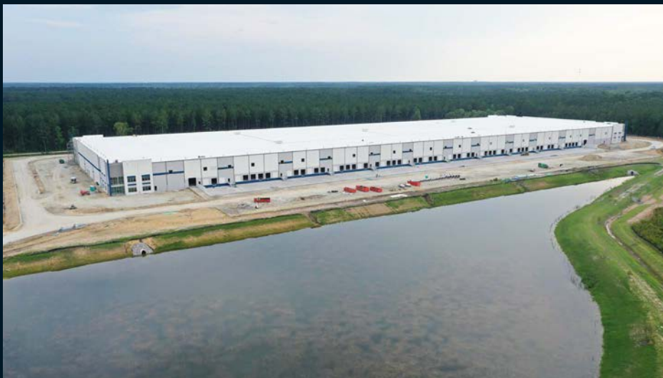
Concrete Truck Court and Drive Aisle
